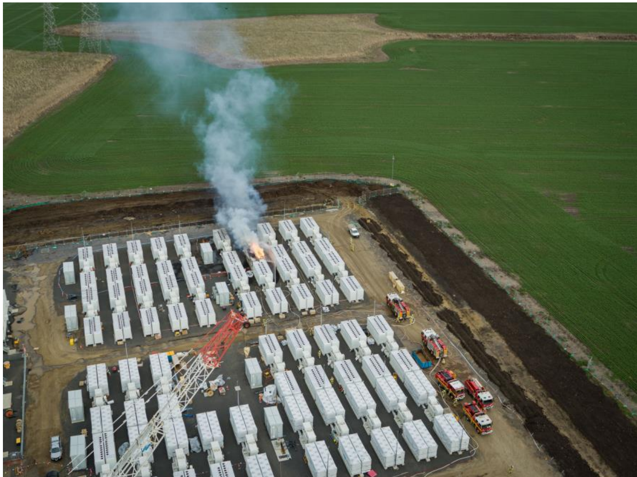
Figure 4 Victoria Big Battery fire incident [47]
