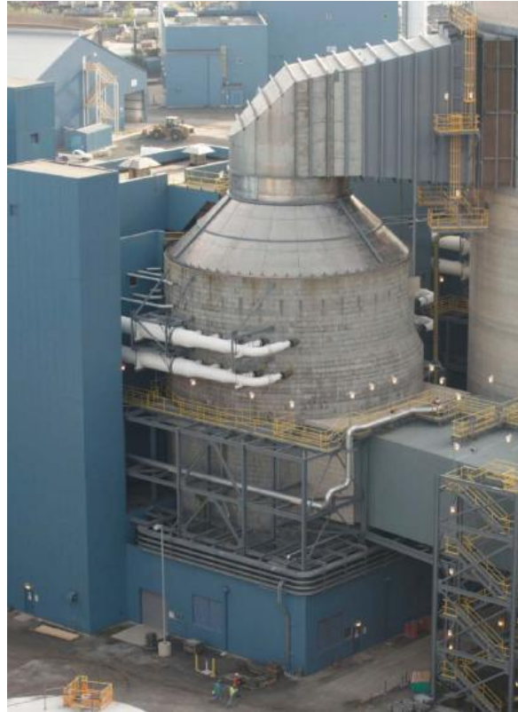
Figure 5.3 Wet FGD System installed at a power plant with one absorber per unit (Babcock & Wilcox, 2012)
