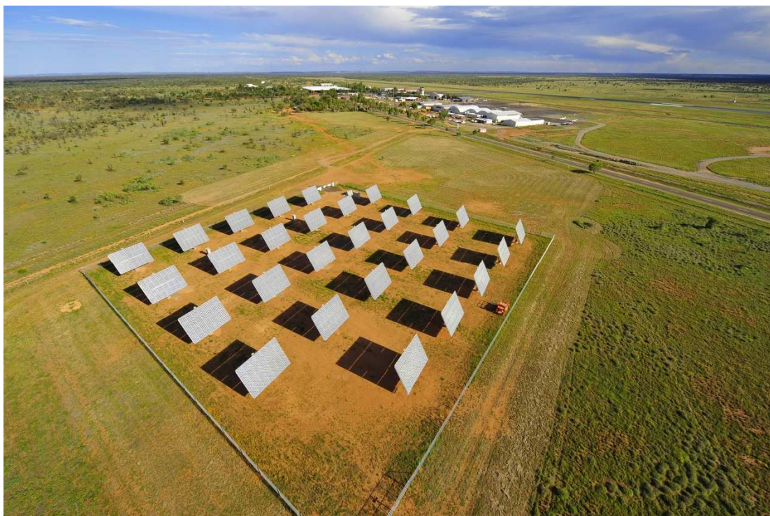
Figure 6 – Alice Springs Airport solar tracking plant
