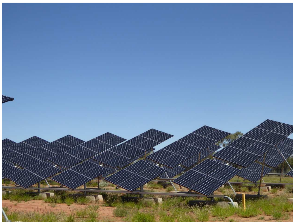
Figure 4 – Uterne Solar Power Station
